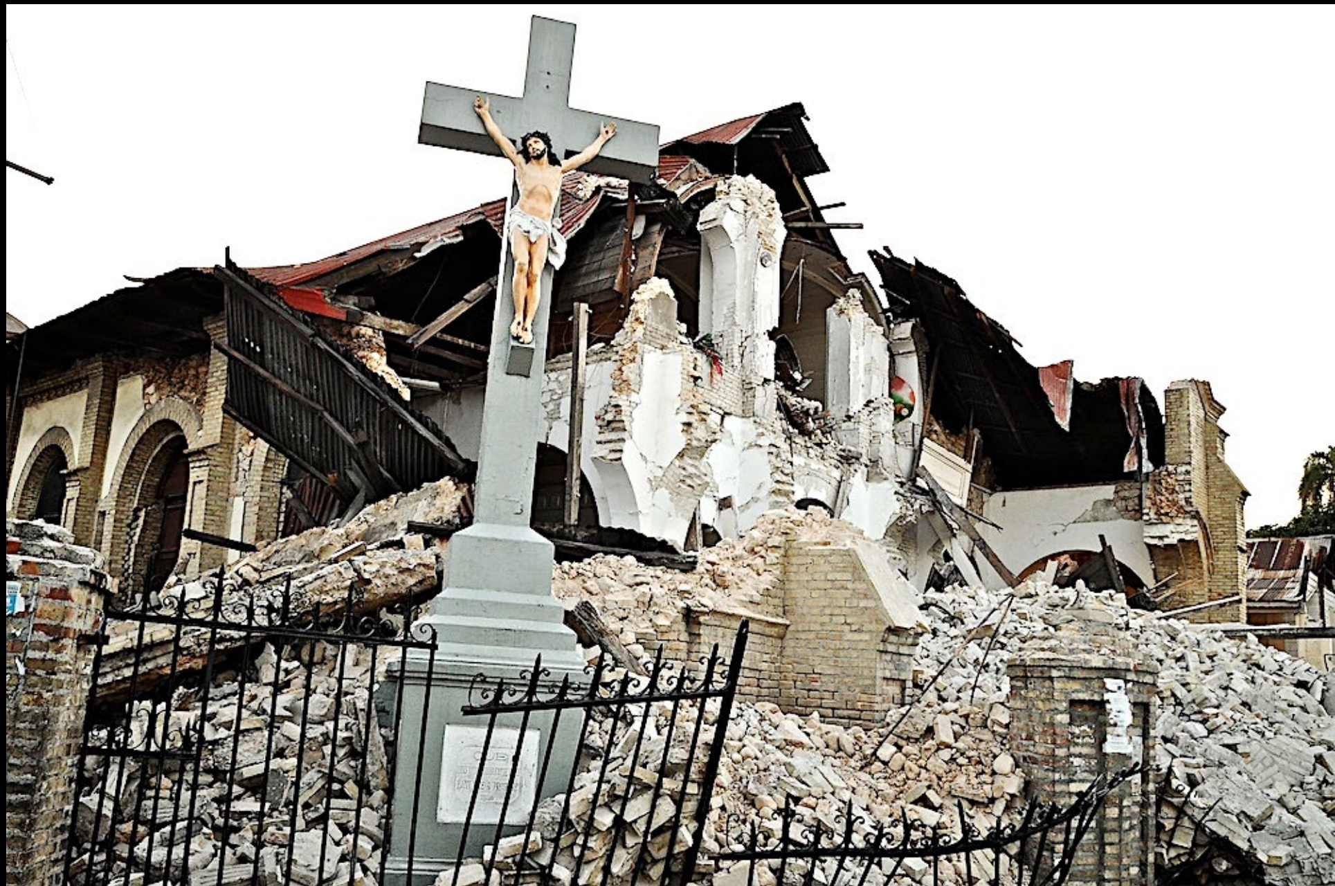
Earthquake Destruction 2010, Port-au-Prince, Haiti
